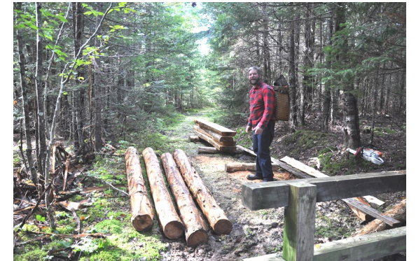
Building bog bridges at Tide Mill Creek.
